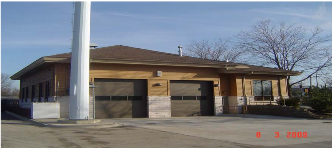
Building Six (Maintenance Shop) 2001 Warrenville Road
